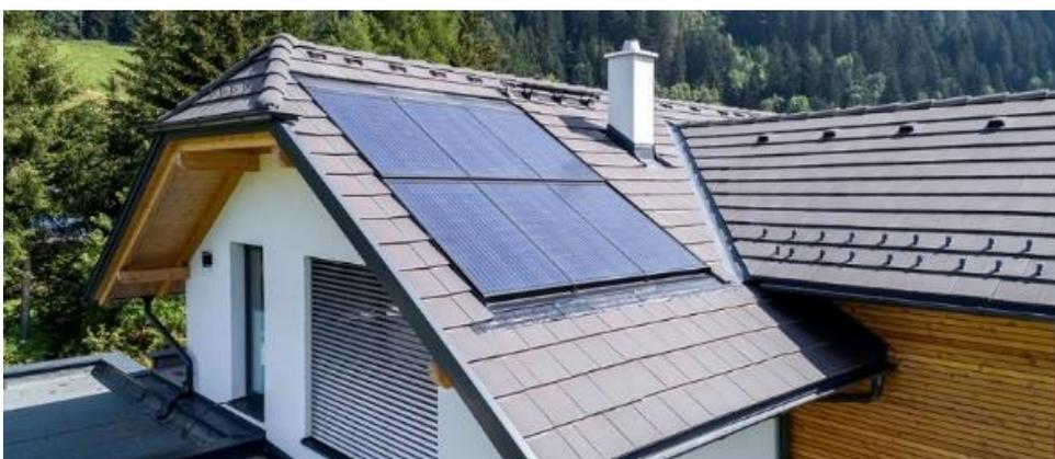
Abbildung 6: Photovoltaik-Indach-System (Quelle: <https://www.bmigroup.com/at/p/pv-modul-bramac-indax-365-half-cut-mono-463164346/?pathname=%2Fat%2Fprodukte%2Fphotovoltaik%2Fphotovoltaik-steildach%2F>) Stand: 25.02.2024
